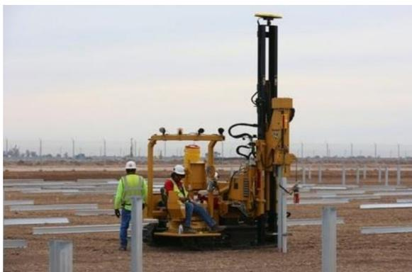
Figure 1 – Hemisphere's heading solution at work (top center), precisely aligning piles for a solar farm installation
